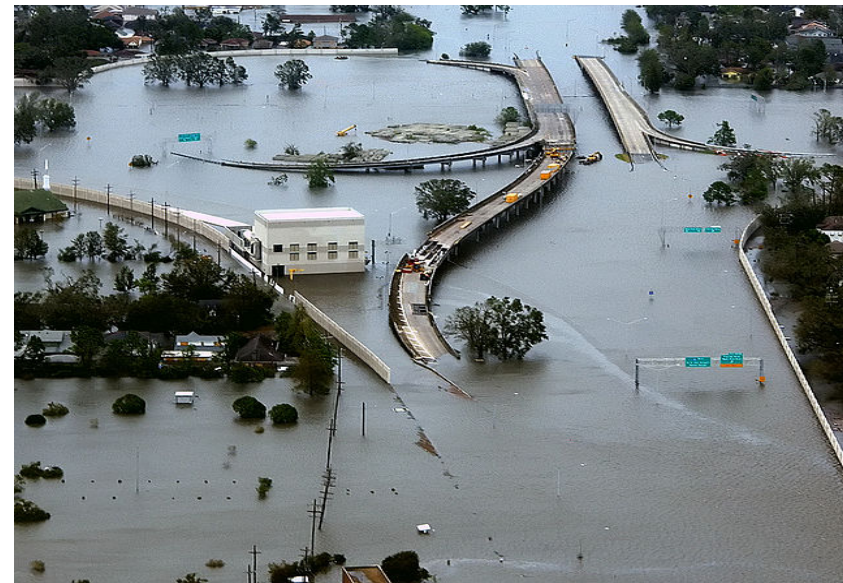
Flooded by storm surge of Hurricane Katrina (2005) in the northwest New Orleans.
