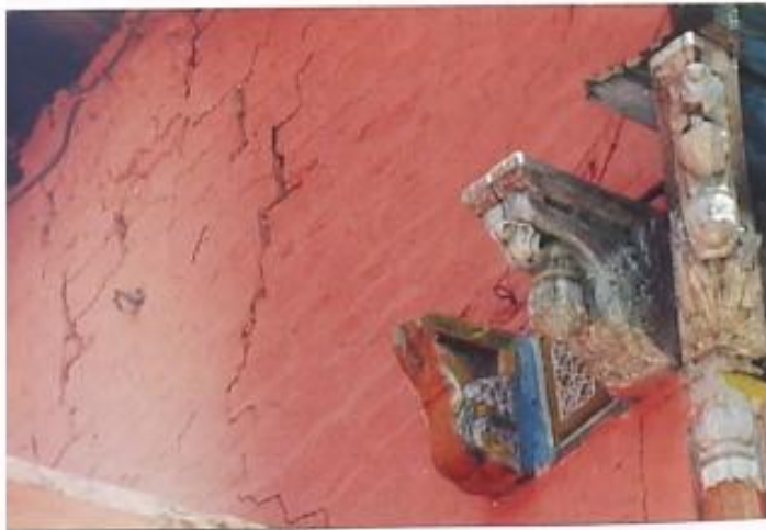
WALL CRACKS
