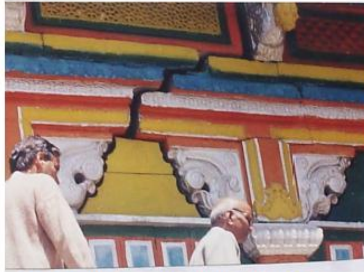
STRUCTURAL CRACKS – BADRINATH TEMPLE FACADE
