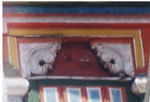
STRUCTURAL CRACKS – BADRINATH TEMPLE FACADE
