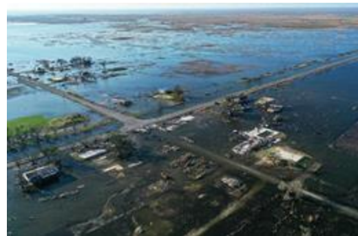
2020 Hurricane Delta causes damage to Louisiana's Gulf Coast
